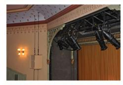
Installing the portable floor monitors was simple, since they could be removed. The mains, however, had to be flown, and had to be easily removable. The solution was to drill four small holes in the auditorium ceiling and install winches to lower the support wires and remove the main speakers as needed, then draw the wires up out of sight.
